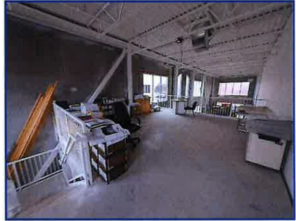
Open Mezzanine Area – View From Front
