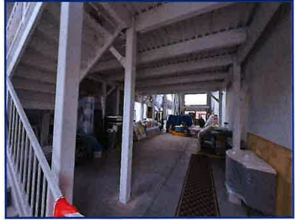
Front Area Under Mezzanine – View From Front
