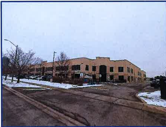
Subject Complex Building A - View from Southeast
