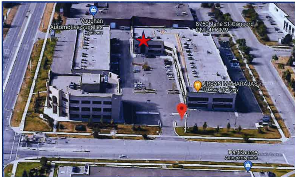
Subject Complex Aerial View - View From North (Gensal Gate)
