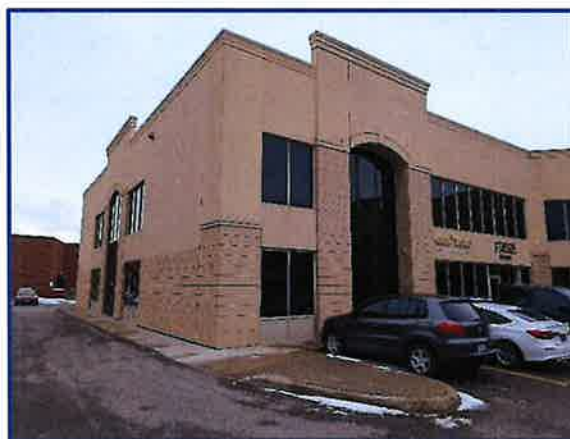
Subject Units - View From Northeast
