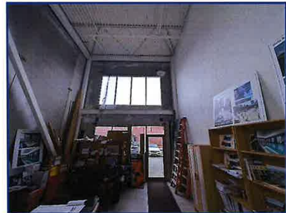
Rear Pedestrian Entrance Door
