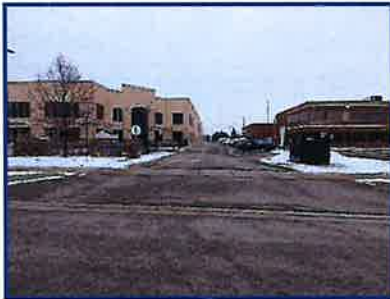
Cut Curb Off Of Romina Drive
