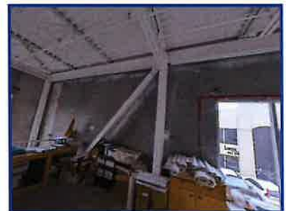
Metal Support Posts and Concrete Curtain Walls
