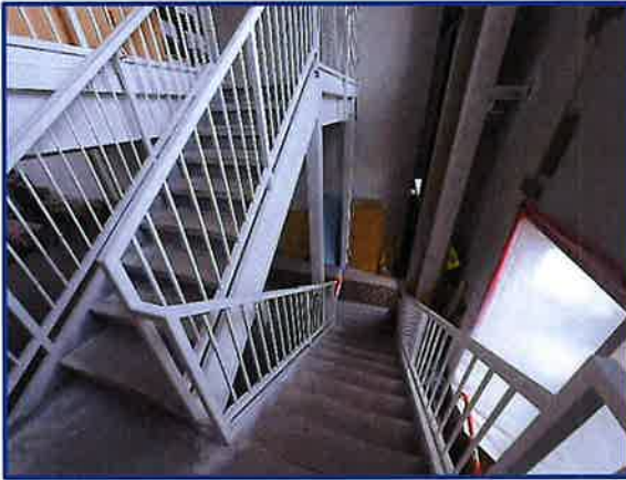
Open Front Stairwell To Mezzanine Level
