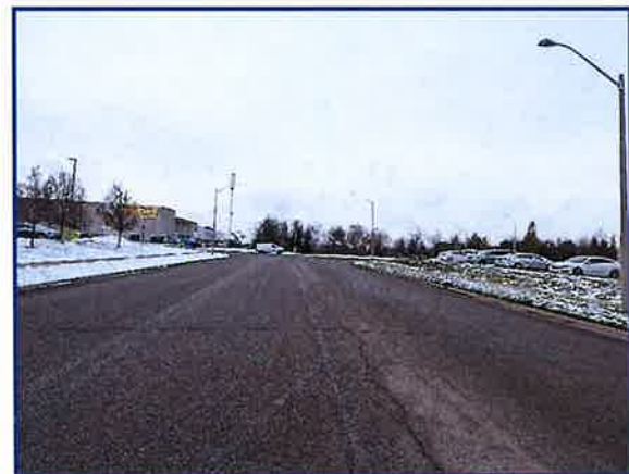
Looking West on Gensal Gate
