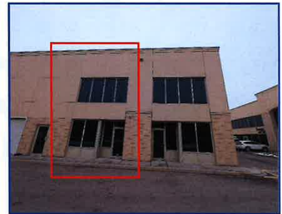
Subject Unit 21 - Rear View
