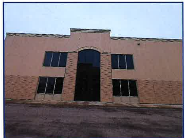
Side Entrance Doors to Unit #22
