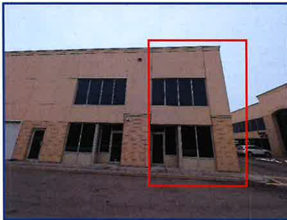
Subject Unit 22 - Rear View
