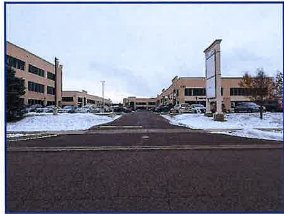
Cut Curb Off Of Gensal Gate
